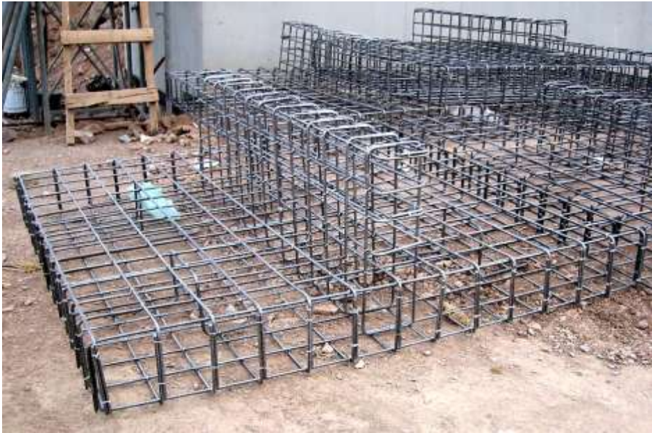
Foundation reinforcement prepared separately.
