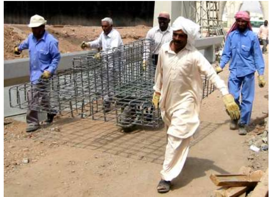
Foundation reinforcement cages transported on site.
