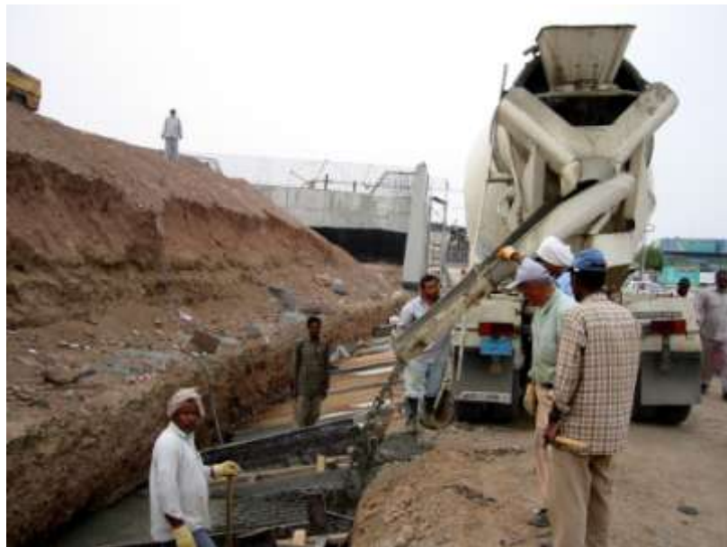
Foundation reinforcement prepared separately.
